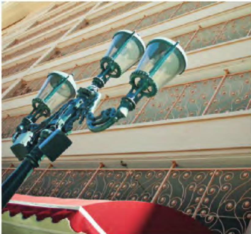
AR Iron and the Venetian Hotel & Casino worked together to make the parking structure at the Vegas attraction safer. The railing had more than 8,000 hand forged half-inch solid bar scrolls, and over 16,000 deco rosettes welded on the finials.
