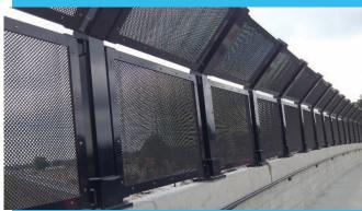
After several data and sample submissions, LEED's recommendation was accepted and the aluminum was coated with a TIGER Drylac Series 38 Super Durable RAL 5004 Deep Blue finish. The company used Nordson Encore guns for powder coating. The end result was a more cost-effective green finish with a performance warranty not offered by the originally specified system.
